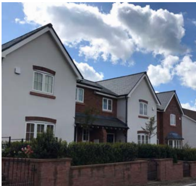
Figure 37: Terraces fronting Wrexham Road.
