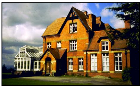
The Beeches built by Joseph Lewis c.1884
