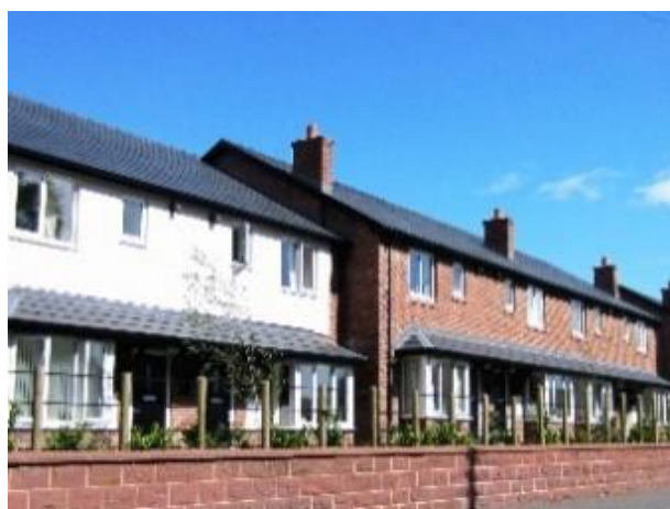
Brockbank (Tilston Road)
