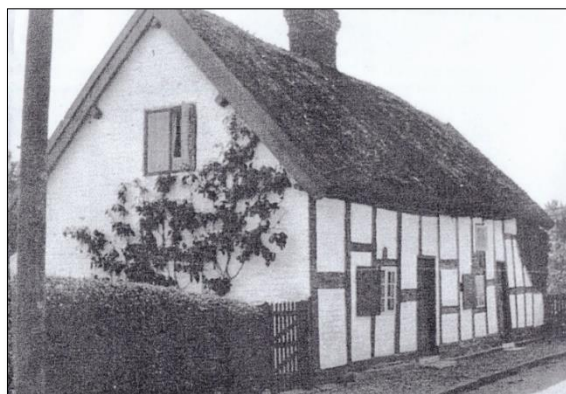
The former Clayholes Cottages
